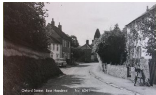
Oxford Street, East Hendred; No. 634; Processed by Fitzwilliams, Seven Kings, Essex
