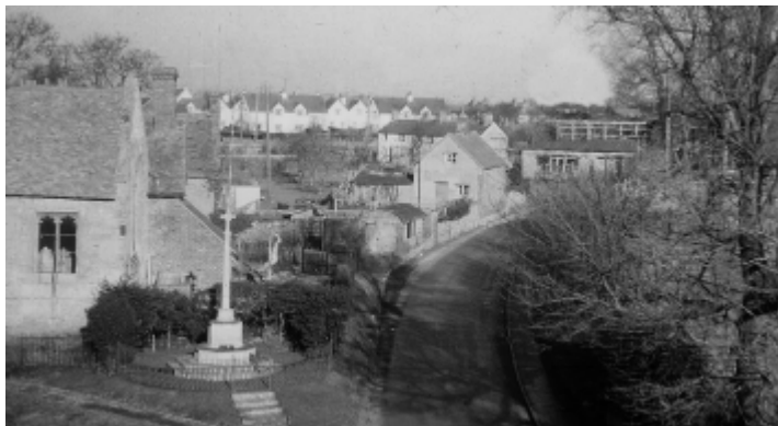
The view north from Champs Chapel to the Spar shop including the pair of cottages to be demolished soon after
